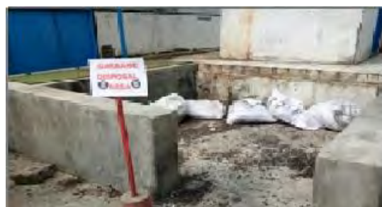
Photo 46) Garbage Disposal area
